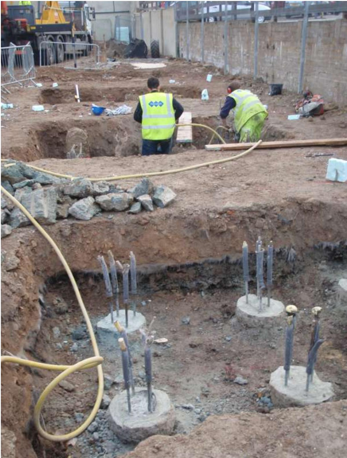
**Plate 3. Phase 2. Ground reduction around pile caps (through made-up ground)**
